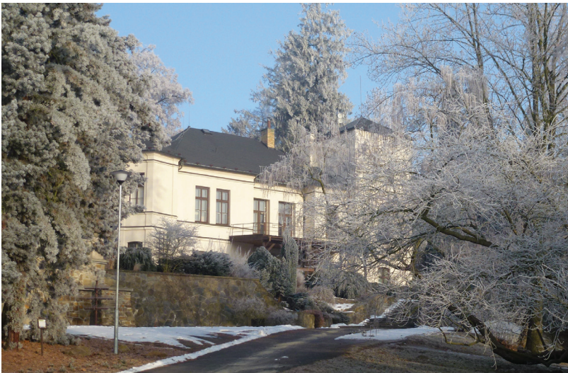
View on historical building – The founder's residence (Můcková, January 2018)
